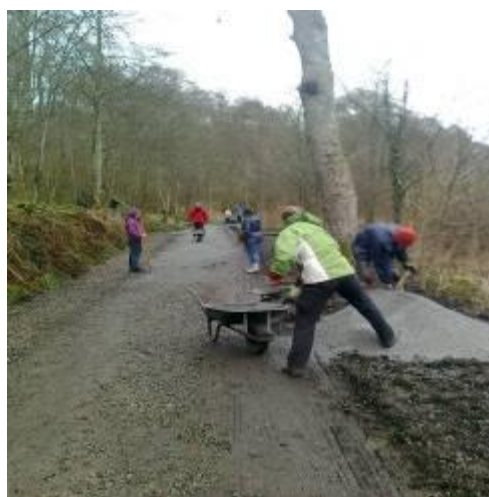
Dirty Weekenders Path Works Photo: Midlothian Ranger Service
