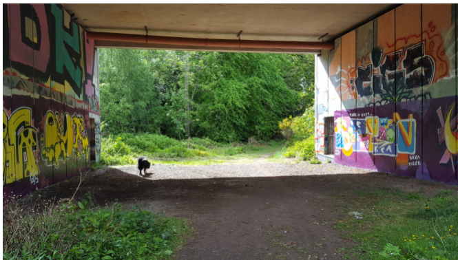
The bridle path off Melville Castle drive, passing under the A7 bridge where graffiti artists practise
